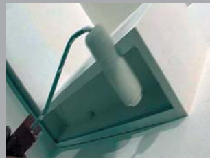
Grinding and coating
